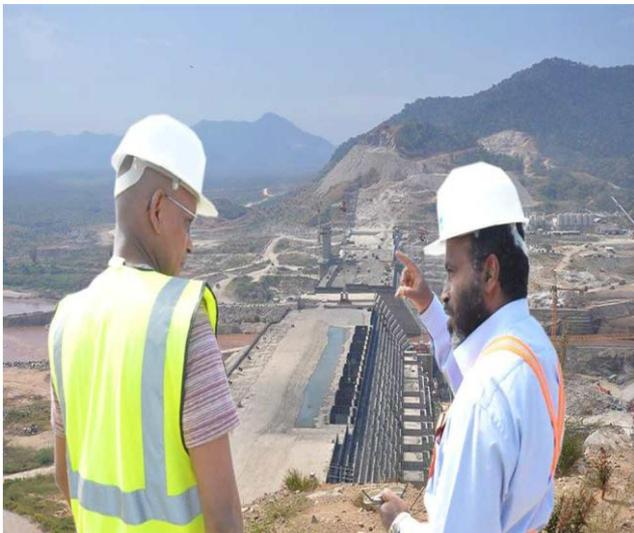
The project includes construction of the main dam in Roller Compacted Concrete (RCC) that is equipped with 21 power stations installed at the foot of the dam. On the other hand, the power stations will have 16 Francis turbines that are equipped with 6000 megawatt and estimated production of 15,700 GWH in a year.
